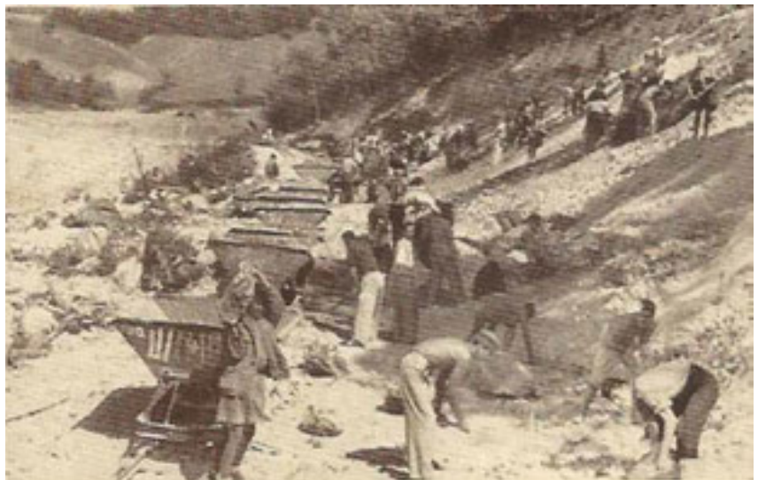
The work on the Šamac – Sarajevo line, 1947.
